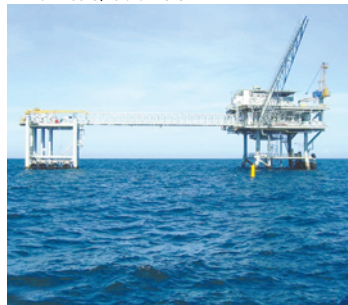
SL60's marking gas transfer lines, Guajira Peninsula, Colombia
